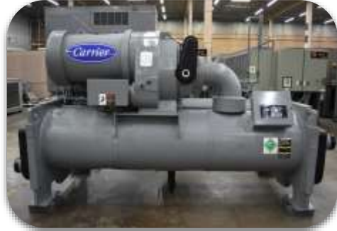
WATER COOLED CHILLED WATER SYSTEM
