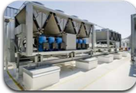
AIR COOLED CHILLED WATER SYSTEM
