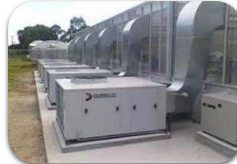
PACKAGE AIR CONDITIONING SYSTEM
